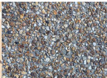
Council standard exposed aggregate concrete paving 'Golden Beach'. Lightly exposed to permit scooter track.
