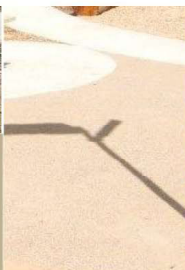
200mm wide concrete edge (top) Council standard coloured concrete paving 'Riverblend Beige'
