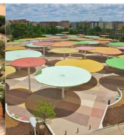
Shelter to have flat, round roof structure with a series of minimal structural posts near the edge. Intention to be non-imposing, non-directional and appear to be a flattened umbrella / parasol as a design cue for the 'weather' in Weatherston.
