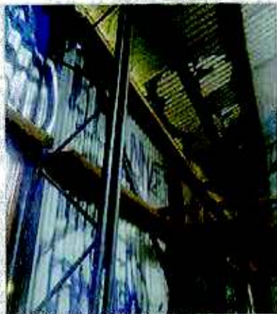
Steel Portal Frame Columns & timber wall girts
