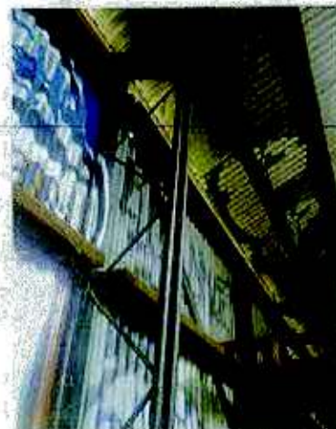
Steel Portal Frame Columns & timber wall girts
