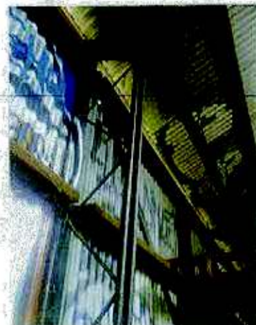
Steel Portal Frame Columns & timber wall girts
