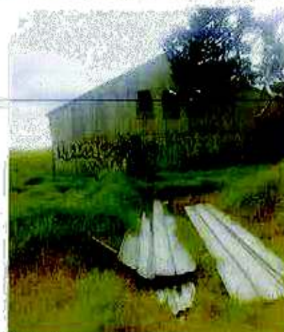
Loose roof sheeting to south side of large shed
