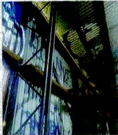
Steel Portal Frame Columns & timber wall girts
